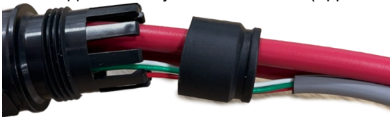
Appendix Figure 2: Grommet prior to inserting into cable gland
